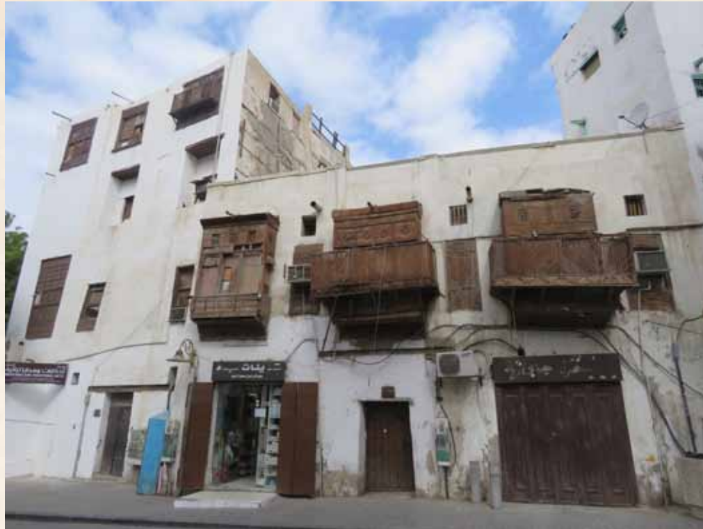
Crown Prince Project to Save and Consolidate the Historic, Archaeologic and National Listed Buildings in Historic Jeddah (56 historic buildings) Bayt Shehata
