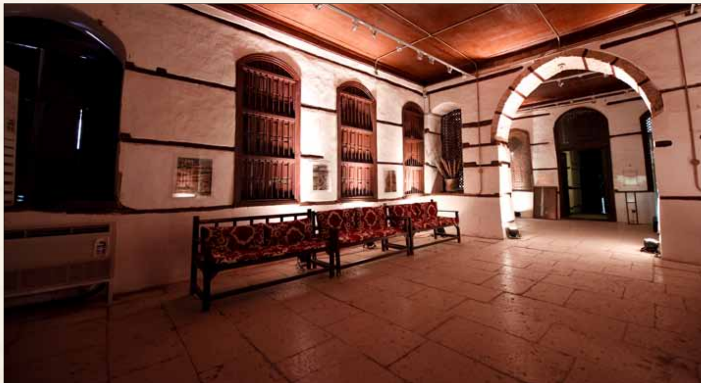
Study, consolidation and restoration of Jeddah's high-risk historic buildings - Bayt Nassif - Historic Jeddah
