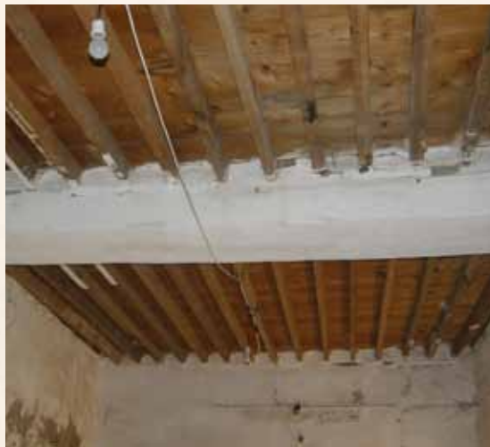
Al-Zawiya Mosque before restoration Al-Madina Al-Munawara
