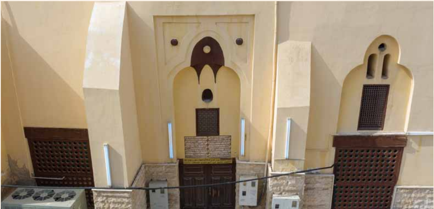
Entrance to Al Hanafi Mosque - Historic Jeddah
