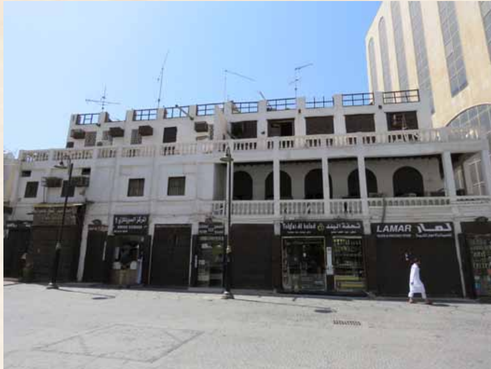
Crown Prince Project to Save and Consolidate the Historic, Archaeologic and National Listed Buildings in Historic Jeddah (56 historic buildings) Bayt Al Amudi Gabel
