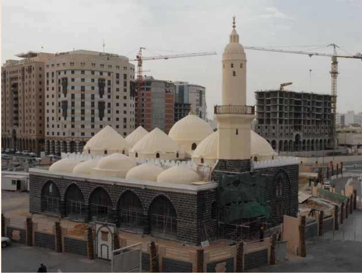
Al-Ghamama Mosque during restoration Al-Madina Al-Munawara
