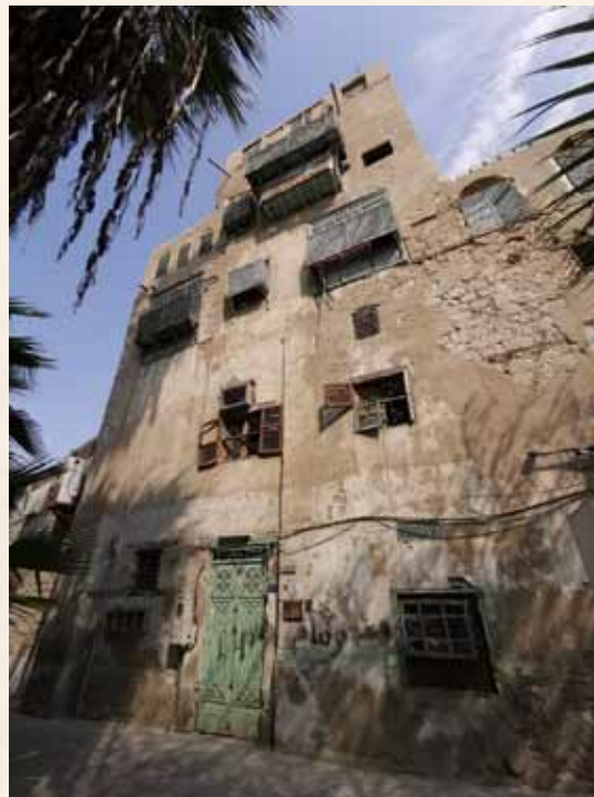
Crown Prince Project to Save and Consolidate the Historic, Archaeologic and National Listed Buildings in Historic Jeddah (56 historic buildings) Bayt Al Khudari
