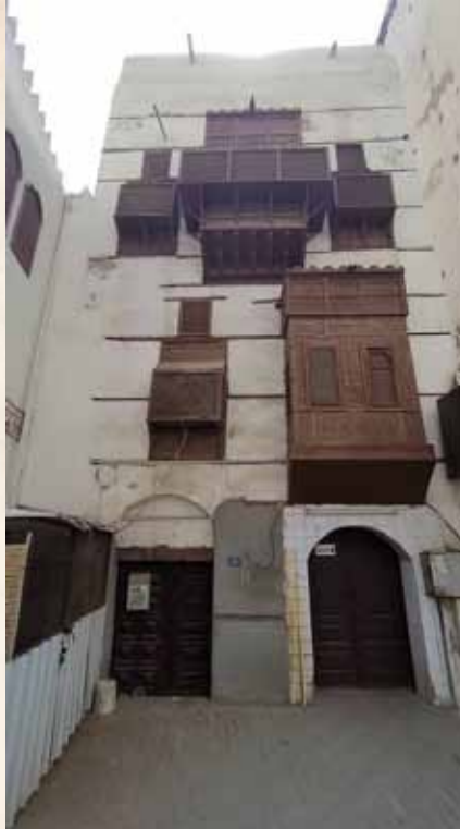
A Project to Prepare a Building Information Modeling System for Historic Buildings (HBIM) in the Historic Jeddah District (For 100 Buildings) N° 1707
