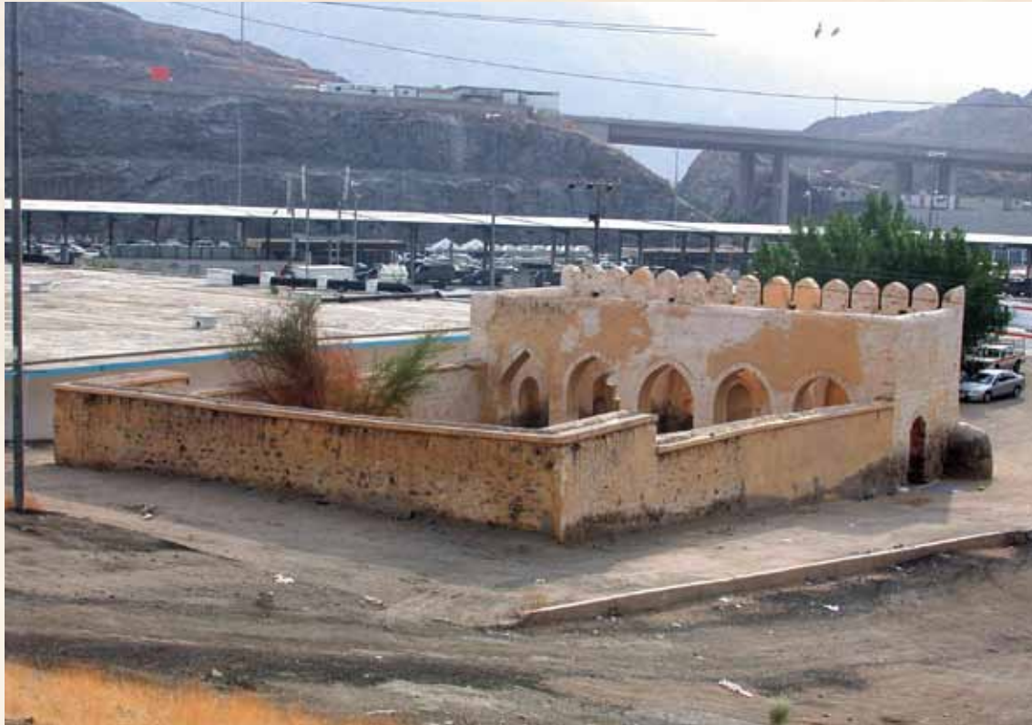
Al-Baiya Mosque before restoration-Makkah Al-Mukarama
