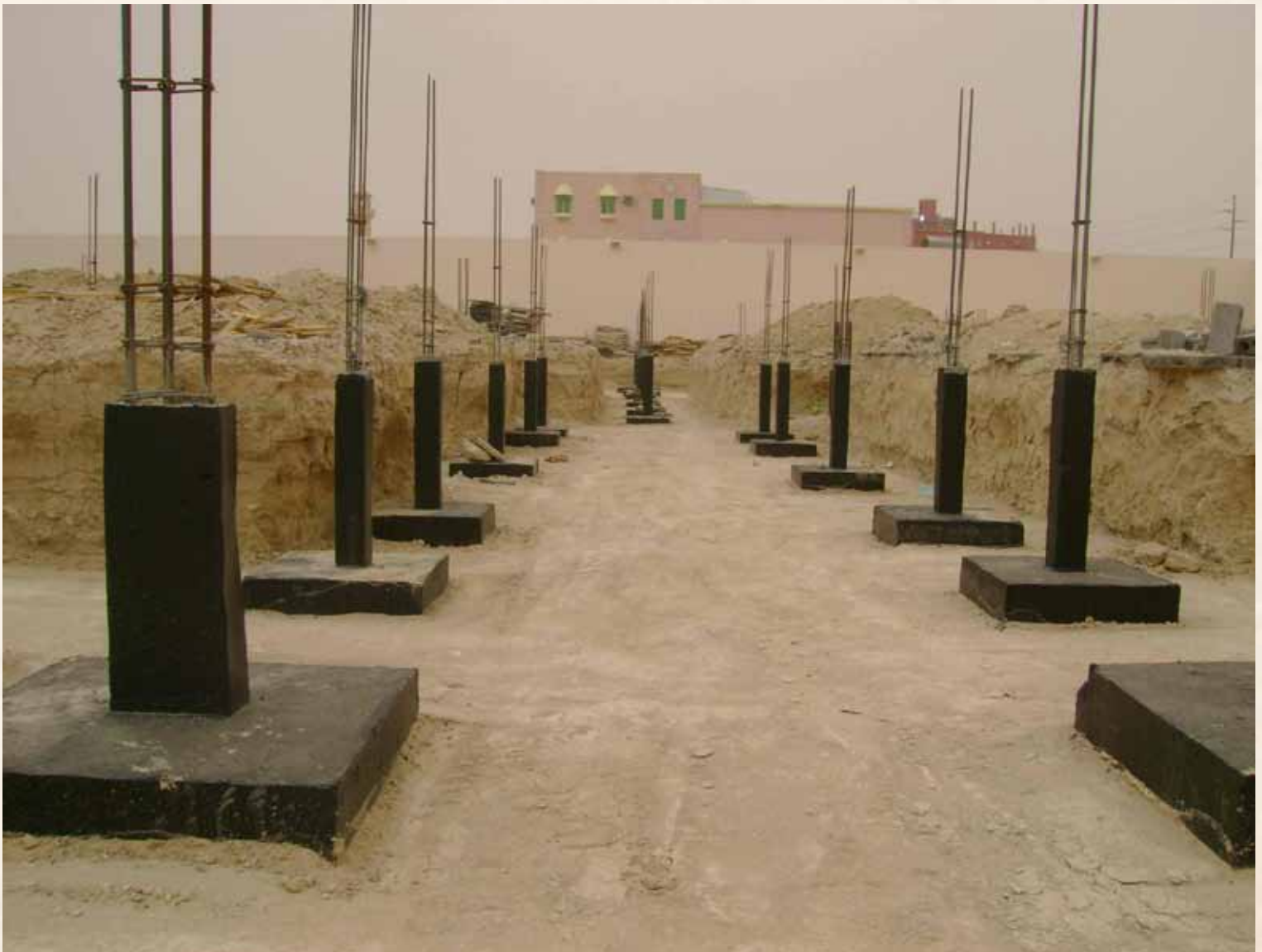
Vocational training center in Al-Ahsa prison during construction - Al Ahsa
