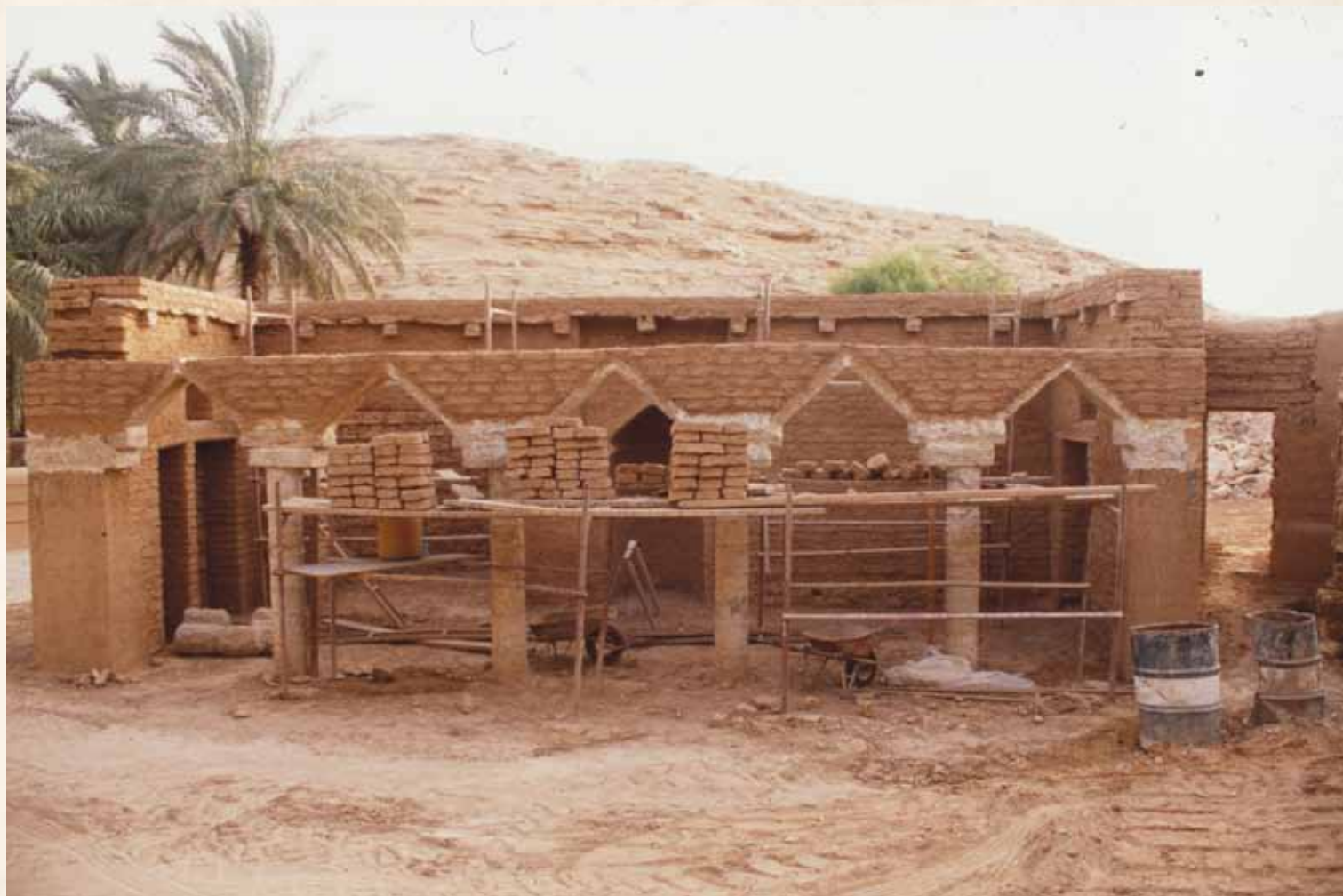
al-'Udhaibāt Mosque during restoration - Historic Ad Diriyah
