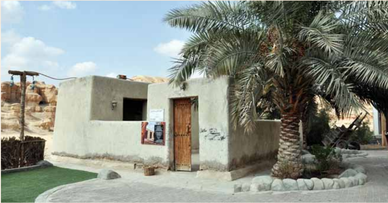
Al-Tahimiyah Mosque (2) before restoration- Al-Tahimiyah
