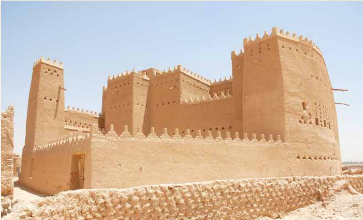
Salwa Palace Compound at Al-Taref District before restoration - Historic Ad Diriyah
