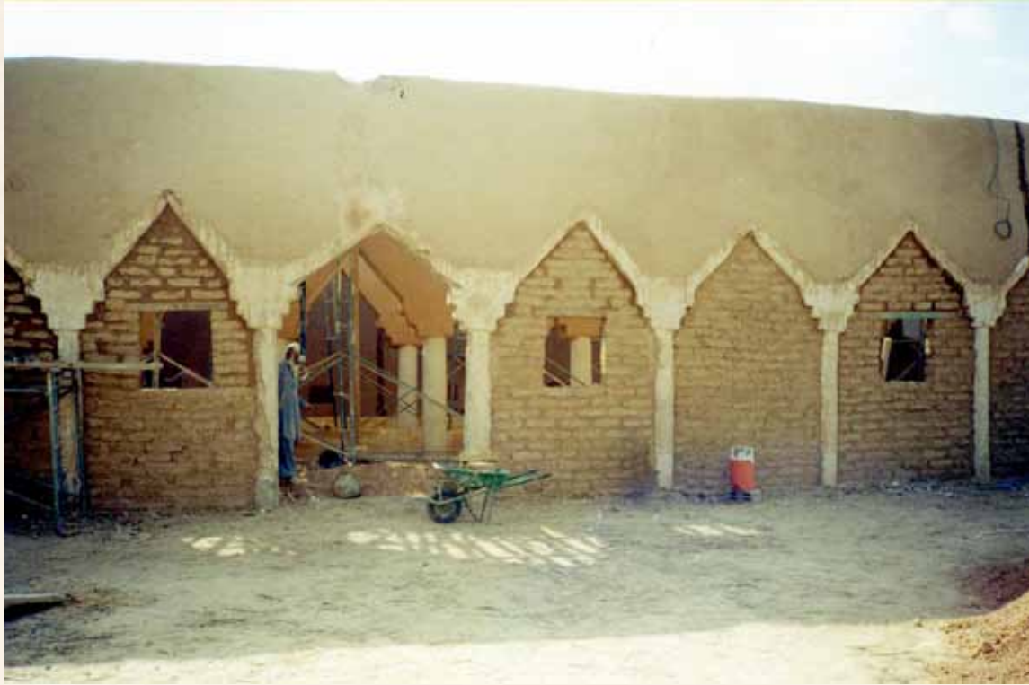
Al-Rmeileh Mosque during the restoration-Arriyadh
