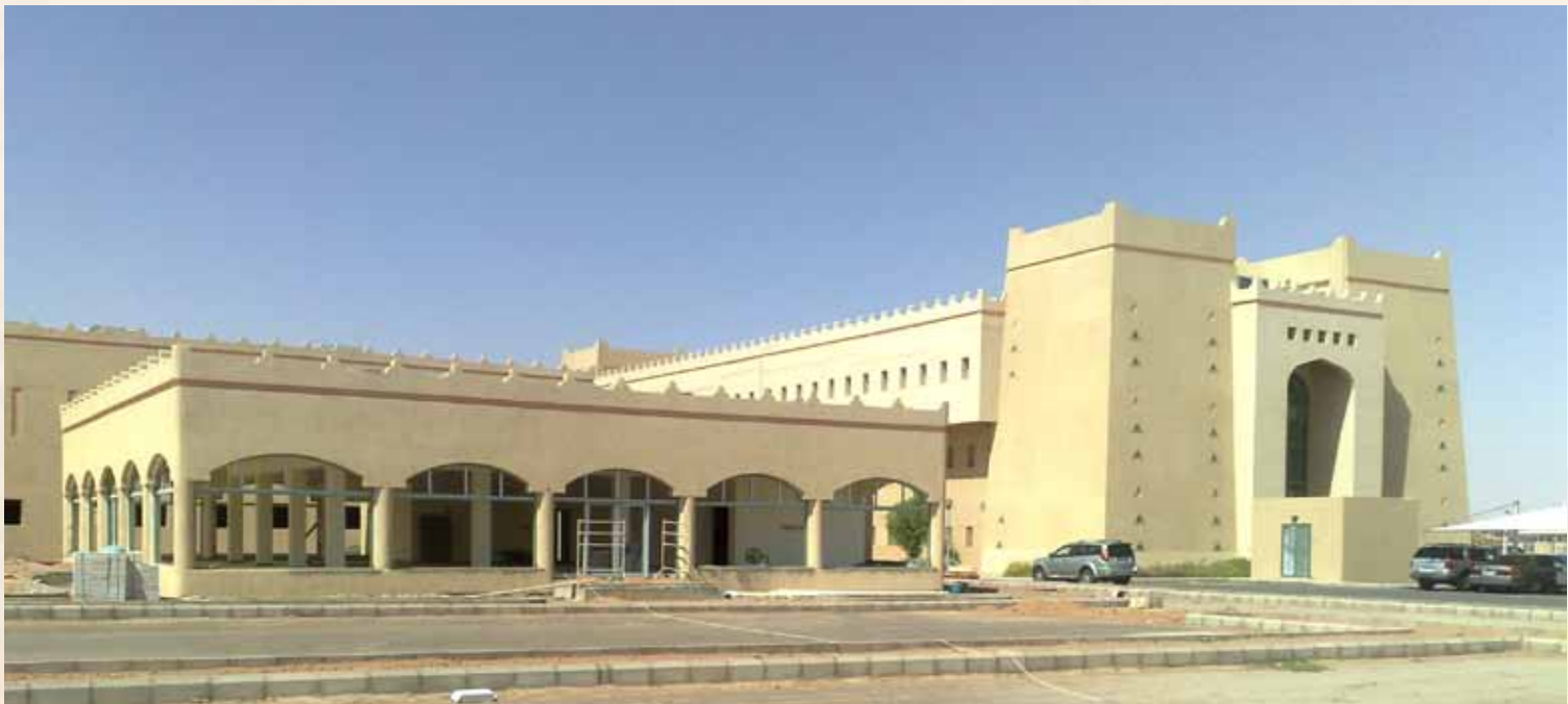
Hail College of Technology - during the completion of the work - Hail
