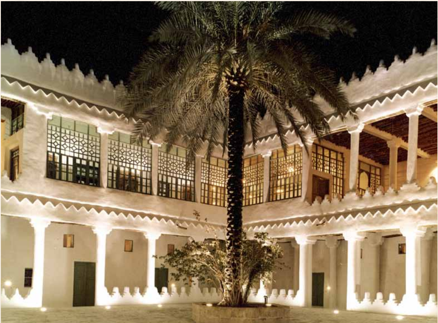
King Abdul-Aziz Palace at Al-Muraba after restoration - Riyadh
