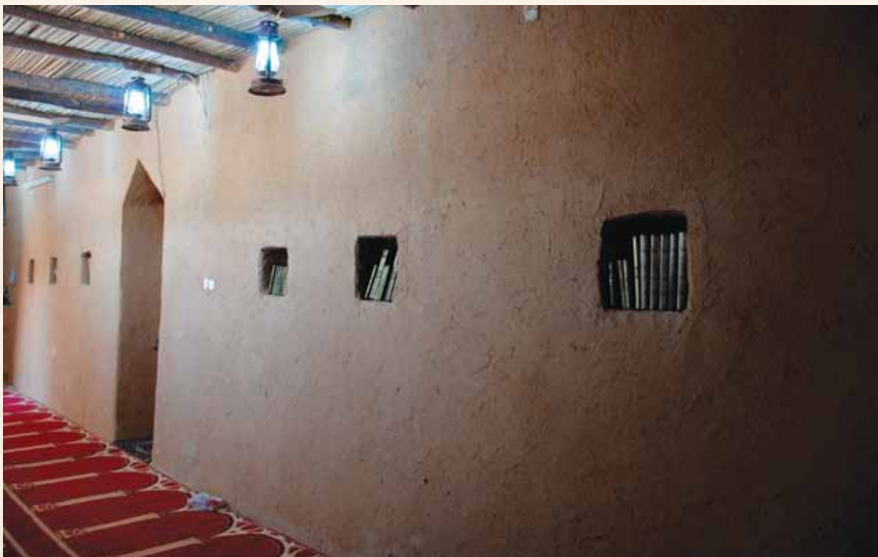
Al-Dawasser Mosque Qibla wall after the last restoration-Historic Ad Diriyah
