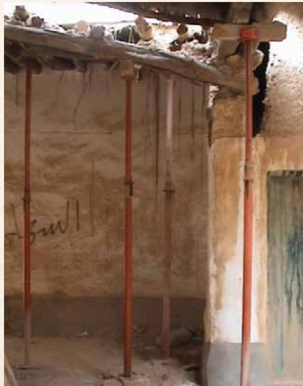
The temporary consolidation of mud installations in the Turaif neighborhood - Historic Ad Diriyah
