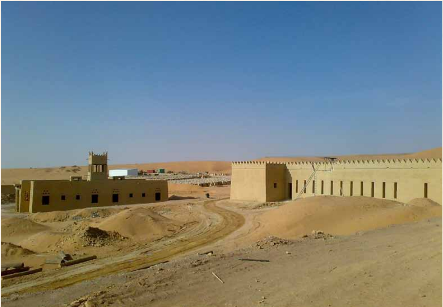
Al-Khalidiya Farm during construction - Riyadh
