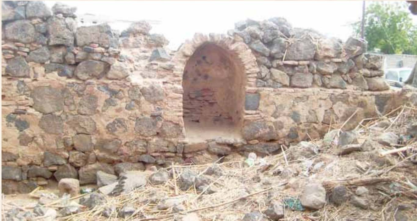
Husseini Mosque from the inside before restoration- Shagra
