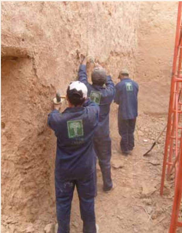
The temporary consolidation of mud installations in the Turaif neighborhood - Historic Ad Diriyah
