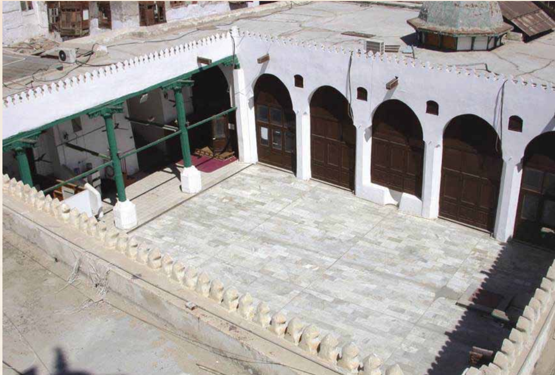
Al-Shafei Mosque before restoration- Historic Jeddah
