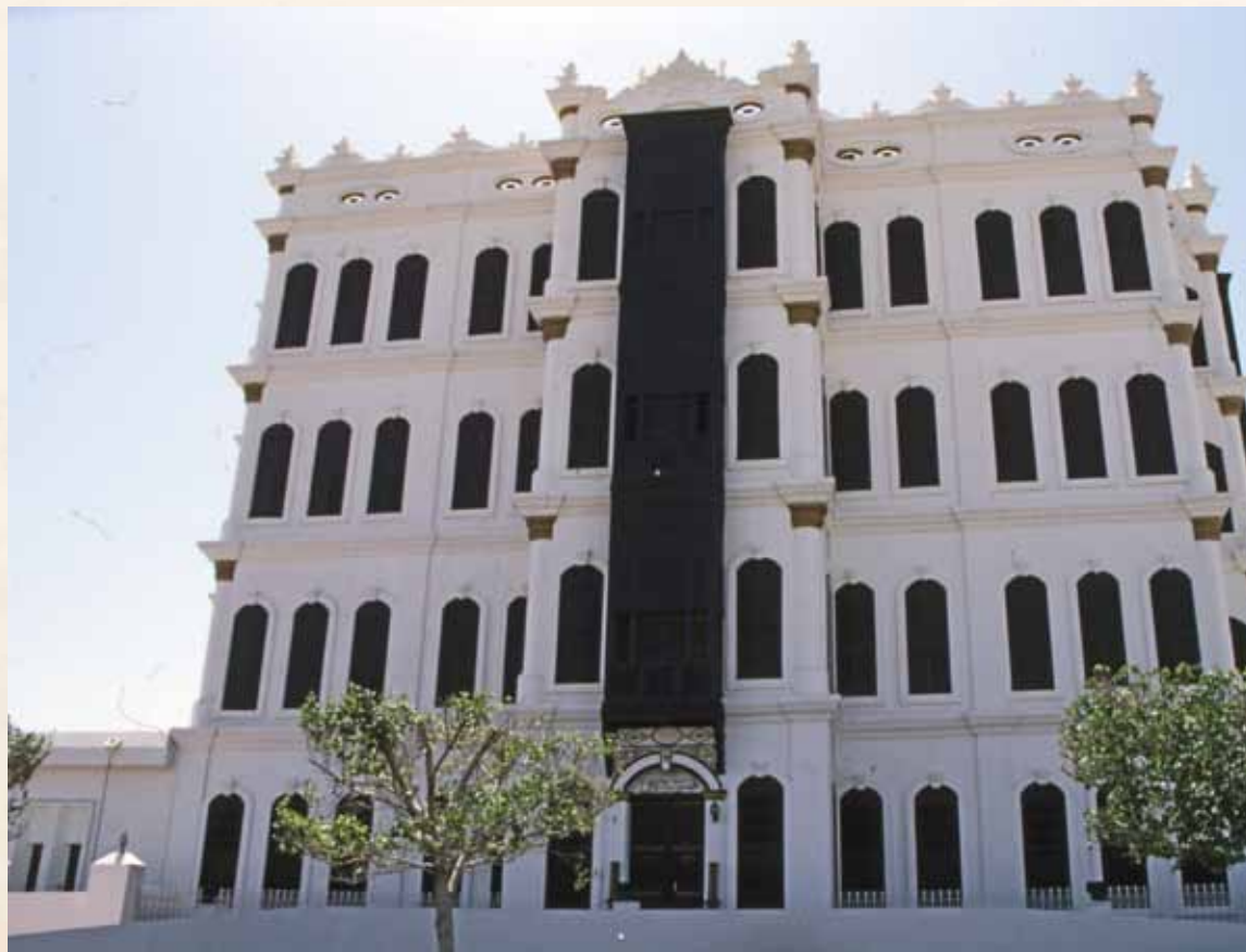
Shubra Historic Palace in Taif after restoration - Taif
