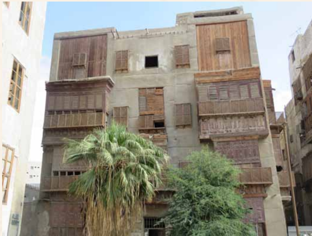
Crown Prince Project to Save and Consolidate the Historic, Archaeologic and National Listed Buildings in Historic Jeddah (56 historic buildings) Bayt Aishmawyi
