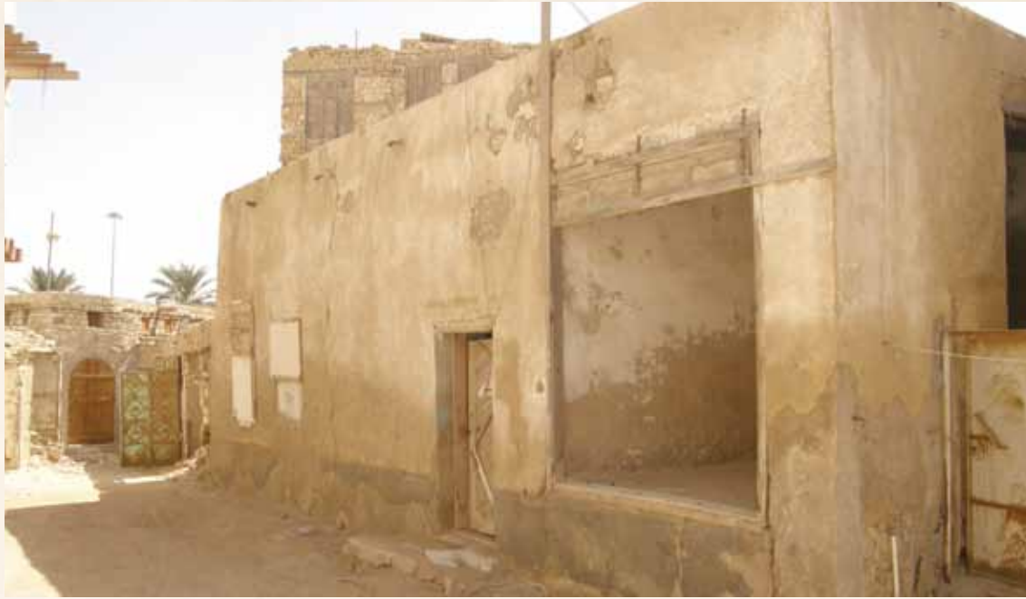
Al-Zawiya Mosque before restoration Al-Madina Al-Munawara
