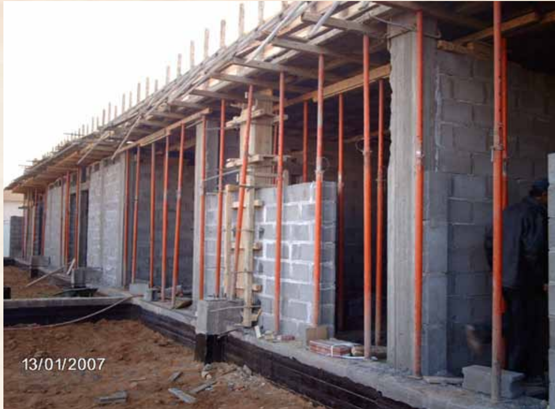
Vocational Training Center in Tabouk Prison during construction works -Tabuk
