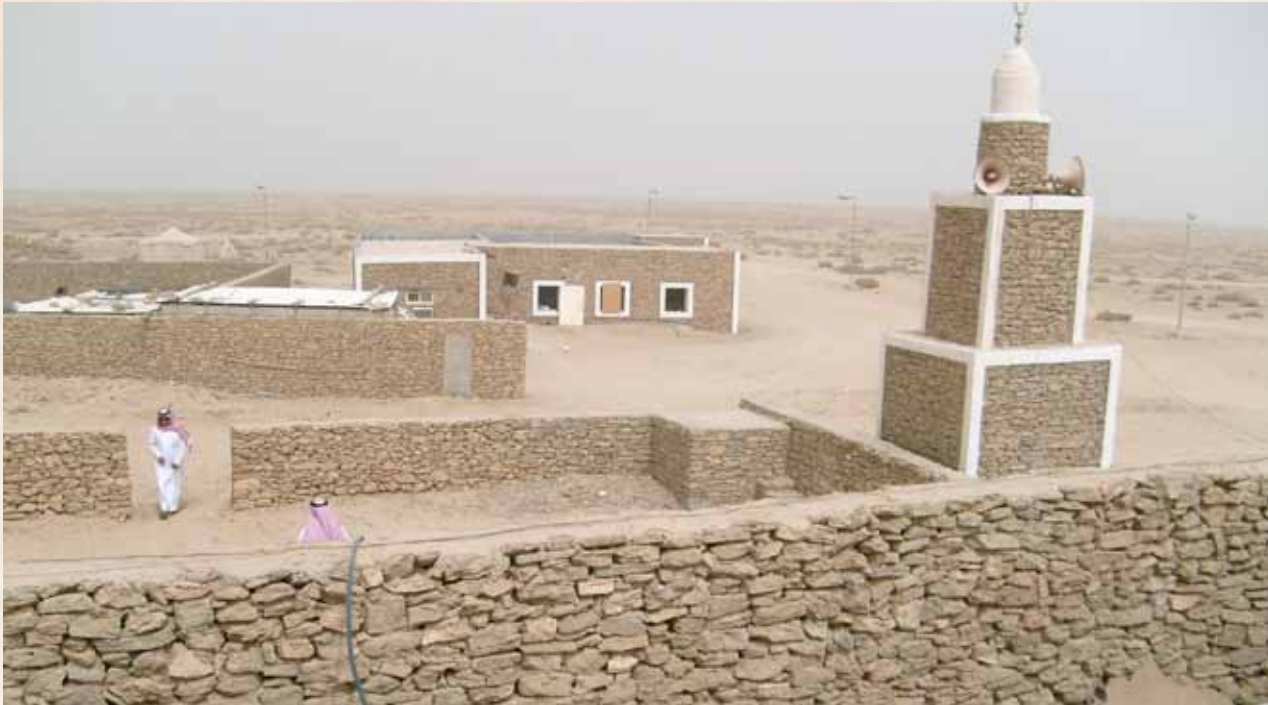
Mosque of Hamad bin Majdal before restoration - Jinna Island, Al Ahsa
