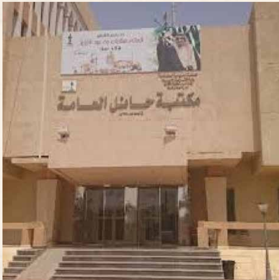
Hail Public Library after restoration -Hail
