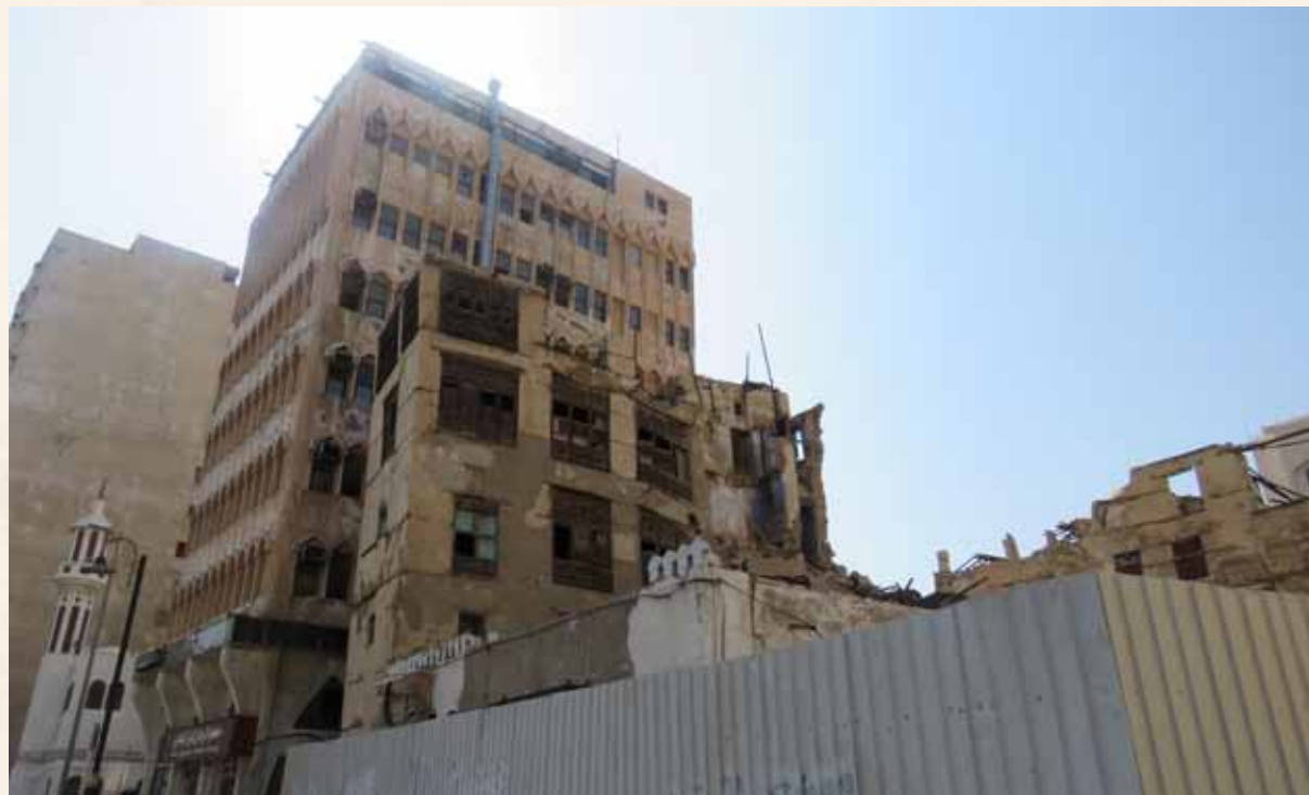
Crown Prince Project to Save and Consolidate the Historic, Archaeologic and National Listed Buildings in Historic Jeddah (56 historic buildings) Bayt Al Mister
