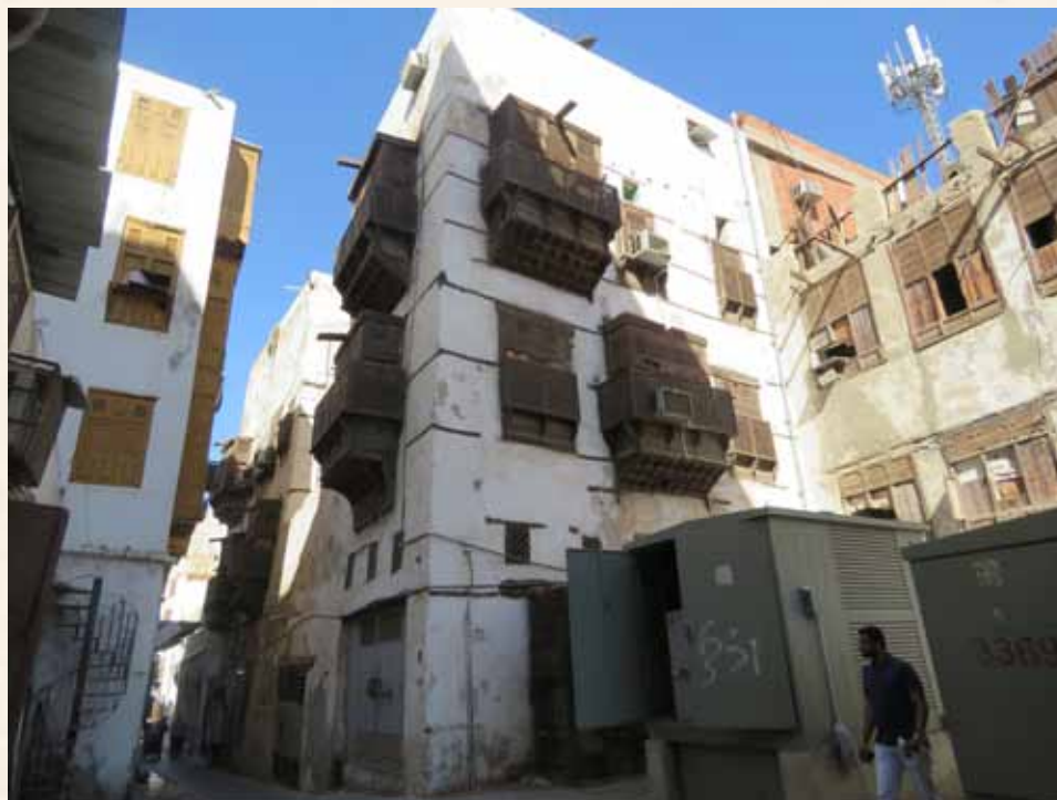
Crown Prince Project to Save and Consolidate the Historic, Archaeologic and National Listed Buildings in Historic Jeddah (56 historic buildings) Bayt Al Timar
