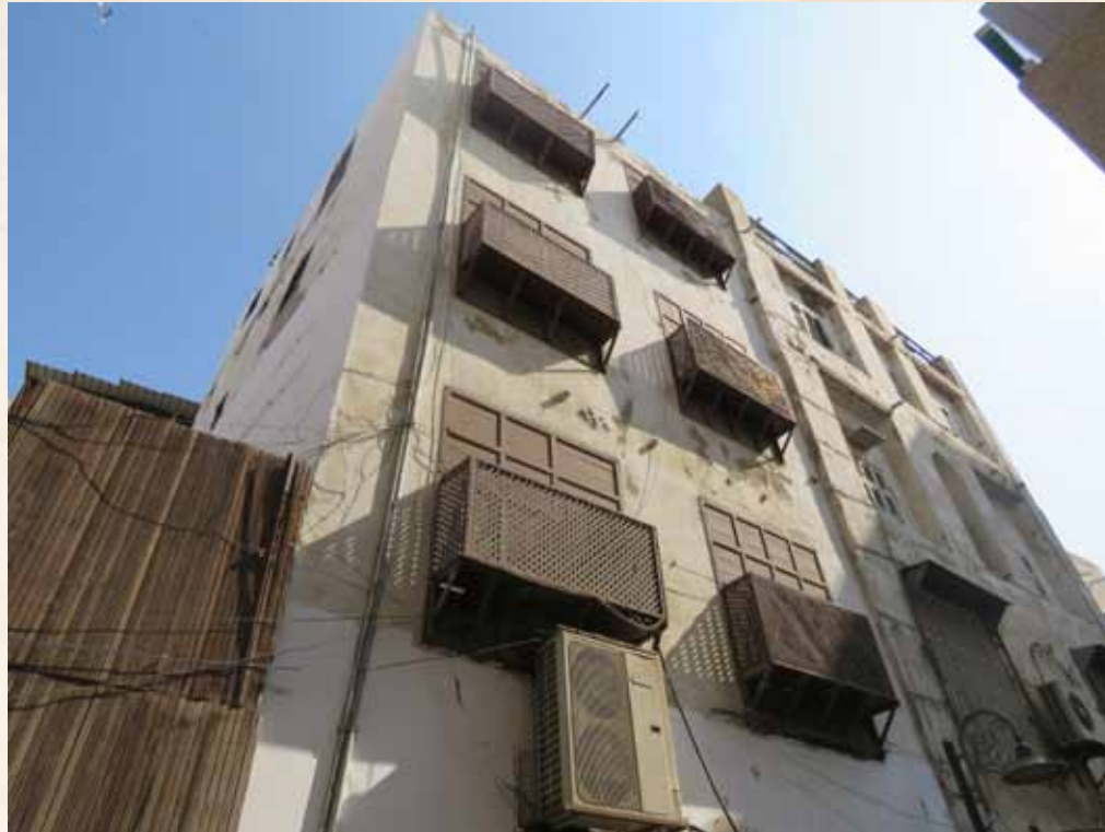
A Project to Prepare a Building Information Modeling System for Historic Buildings (HBIM) in the Historic Jeddah District (For 100 Buildings) Bayt Gandel
