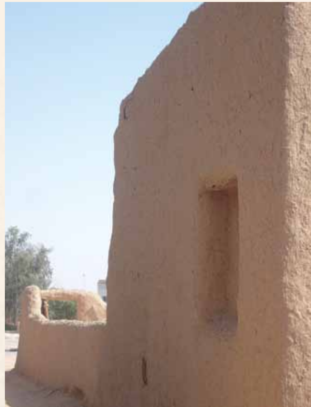
Side facade of Qerasha Mosque - Huraymala
