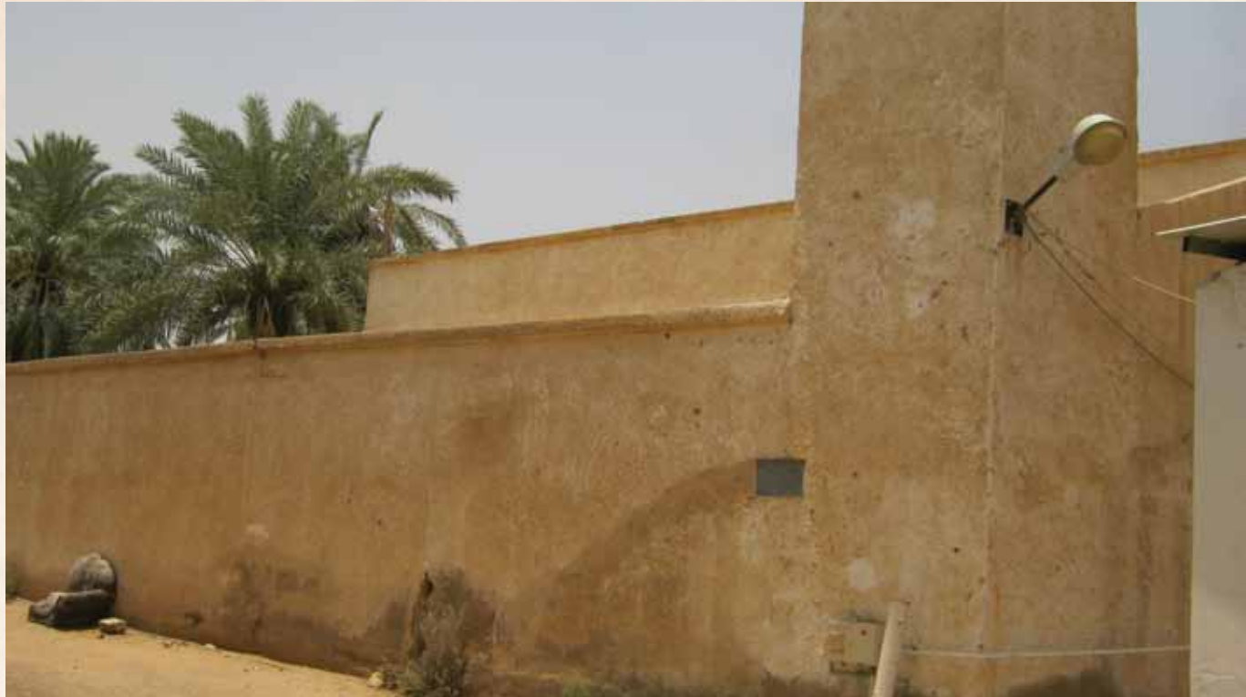
Al Murih Mosque before restoration- Arriyadh
