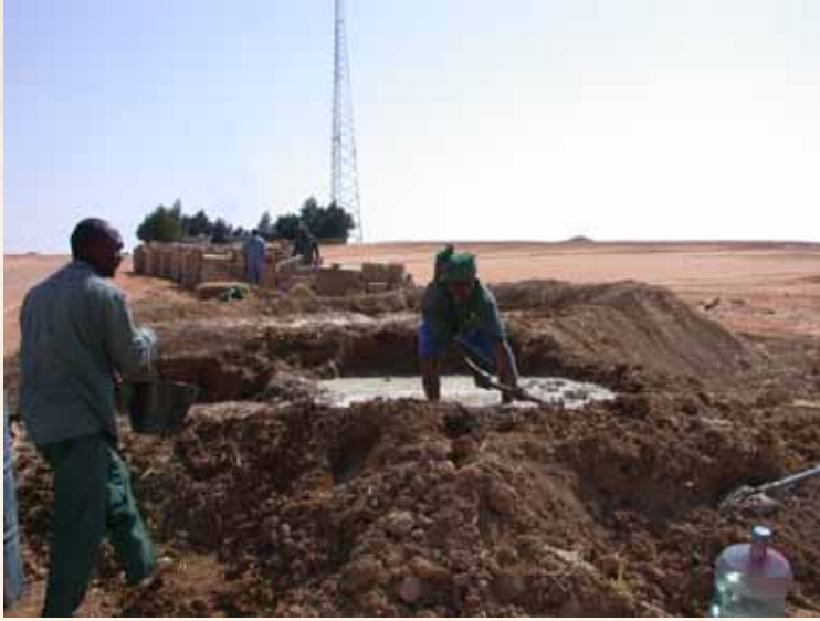
During the preparation of Mud - Riyadh
