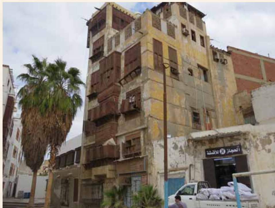
Crown Prince Project to Save and Consolidate the Historic, Archaeologic and National Listed Buildings in Historic Jeddah (56 historic buildings) Waqaf Falah
