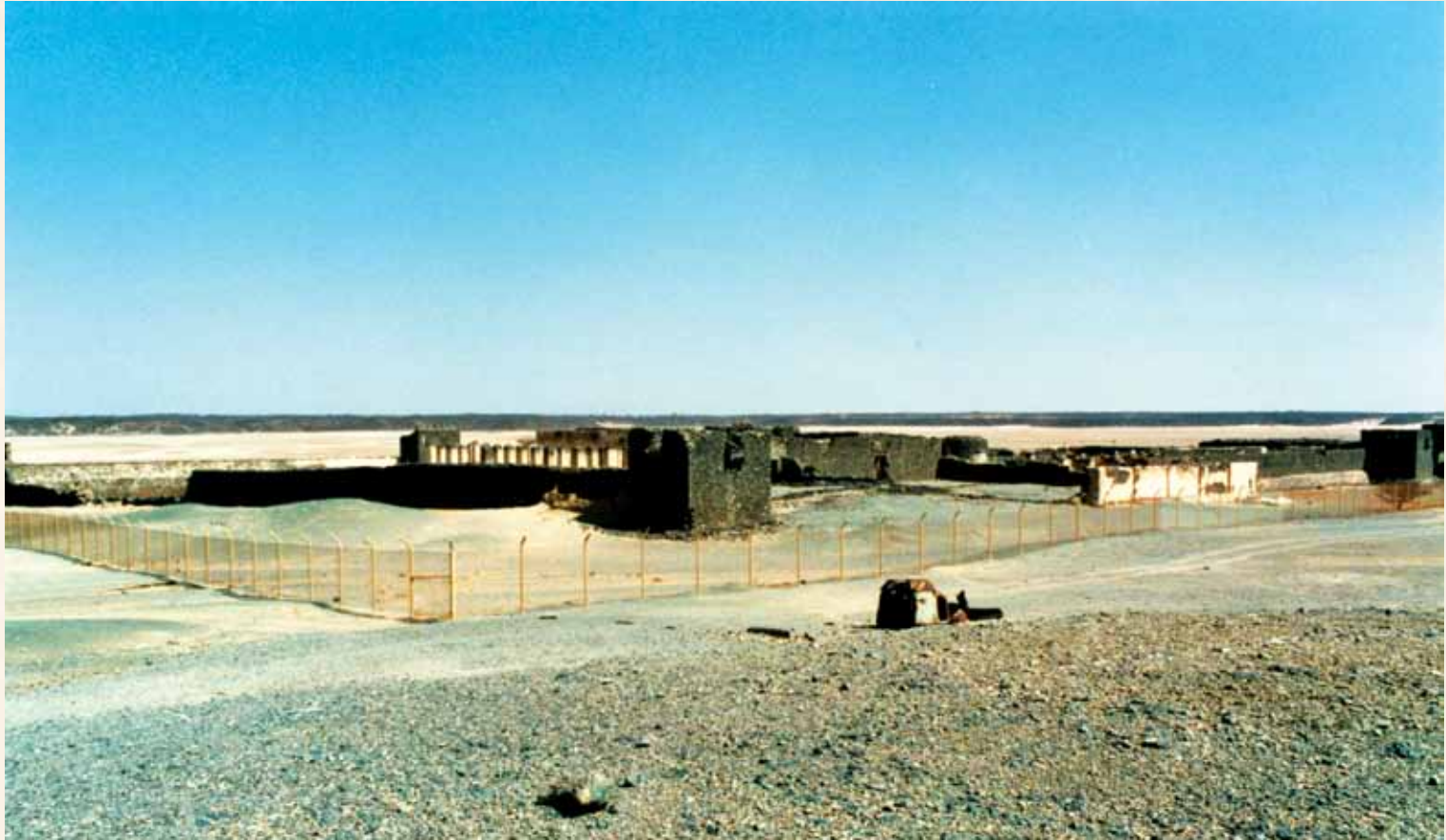
King Abdul-Aziz Palace before the restoration and during the preparation of studies - Al-Muwayh
