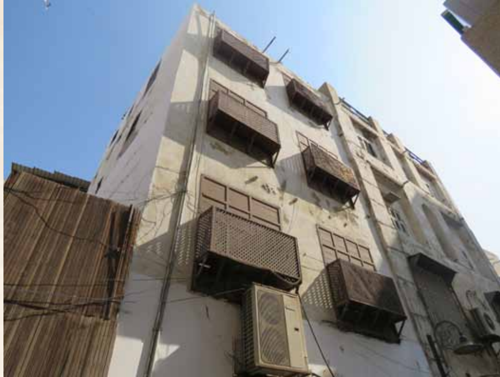
Crown Prince Project to Save and Consolidate the Historic, Archaeologic and National Listed Buildings in Historic Jeddah (56 historic buildings) Bayt Gandel
