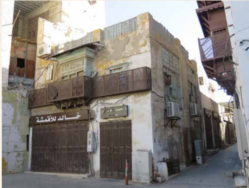
Crown Prince Project to Save and Consolidate the Historic, Archaeologic and National Listed Buildings in Historic Jeddah (56 historic buildings) Bayt Al Halawani
