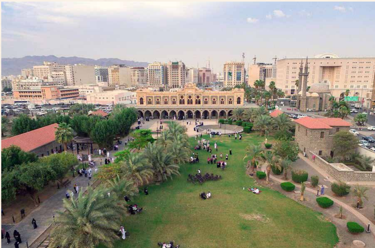
The main building of the Hijaz Railway station after restoration - Al-Madina Al-Munawara
