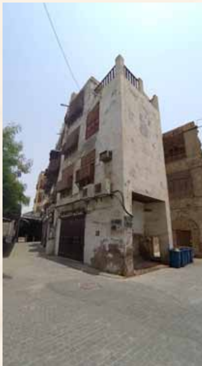
A Project to Prepare a Building Information Modeling System for Historic Buildings (HBIM) in the Historic Jeddah District (For 100 Buildings) N° 1757
