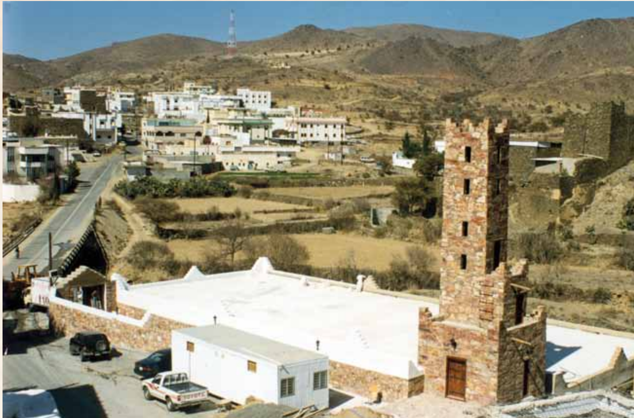
Imam Saud bin Abdulaziz bin Mohammed Mosque before restoration-Tabab
