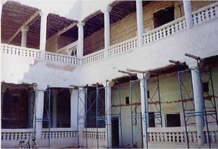
King Abdul-Aziz Palace at Al-Muraba during restoration -Riyadh
