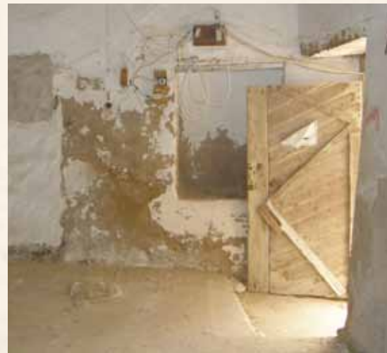
Al-Zawiya Mosque before restoration Al-Madina Al-Munawara
