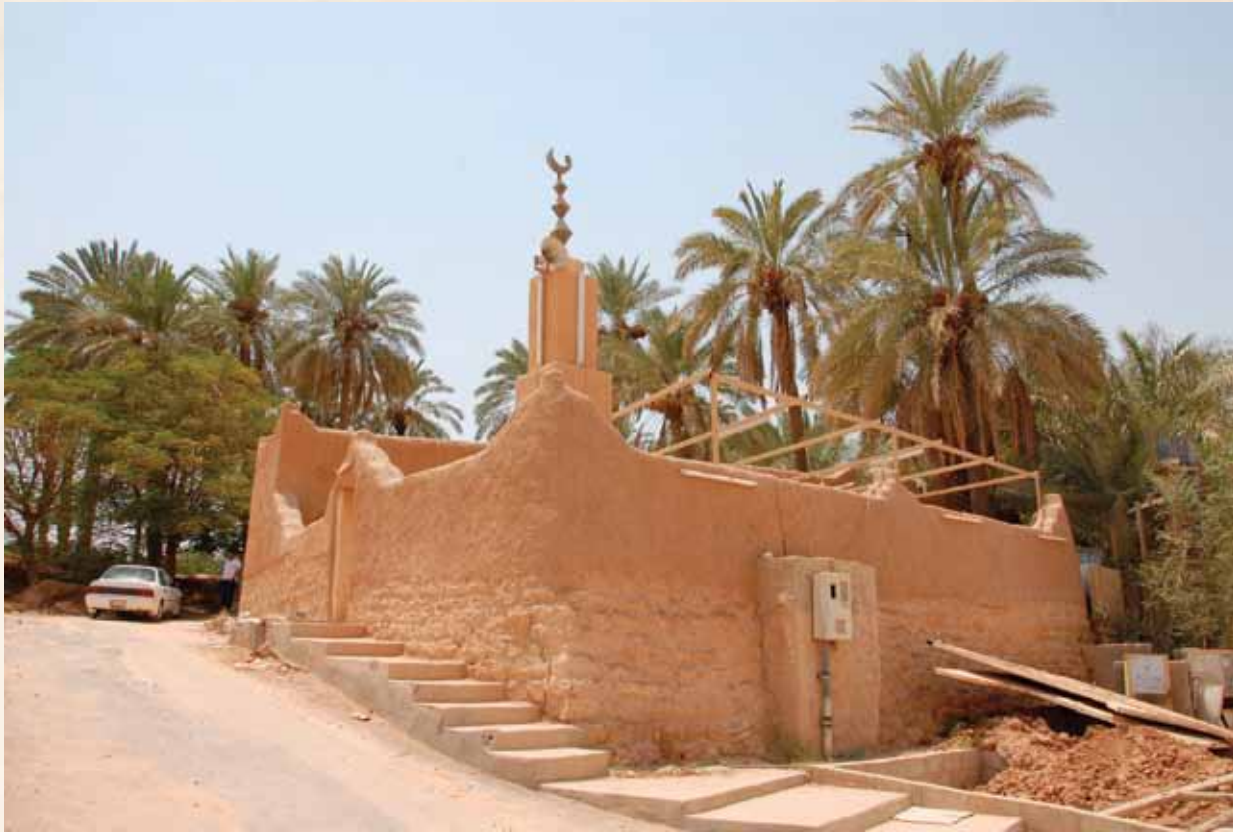
Al-Dawasser Mosque before restoration-Historic Ad Diriyah
