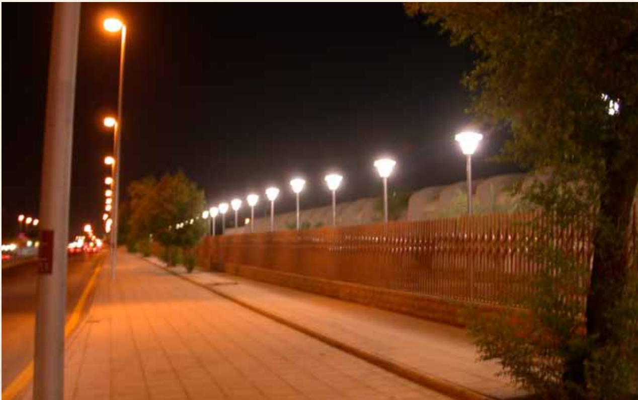
Modern Institute of the Capital after development work - Arriyadh
