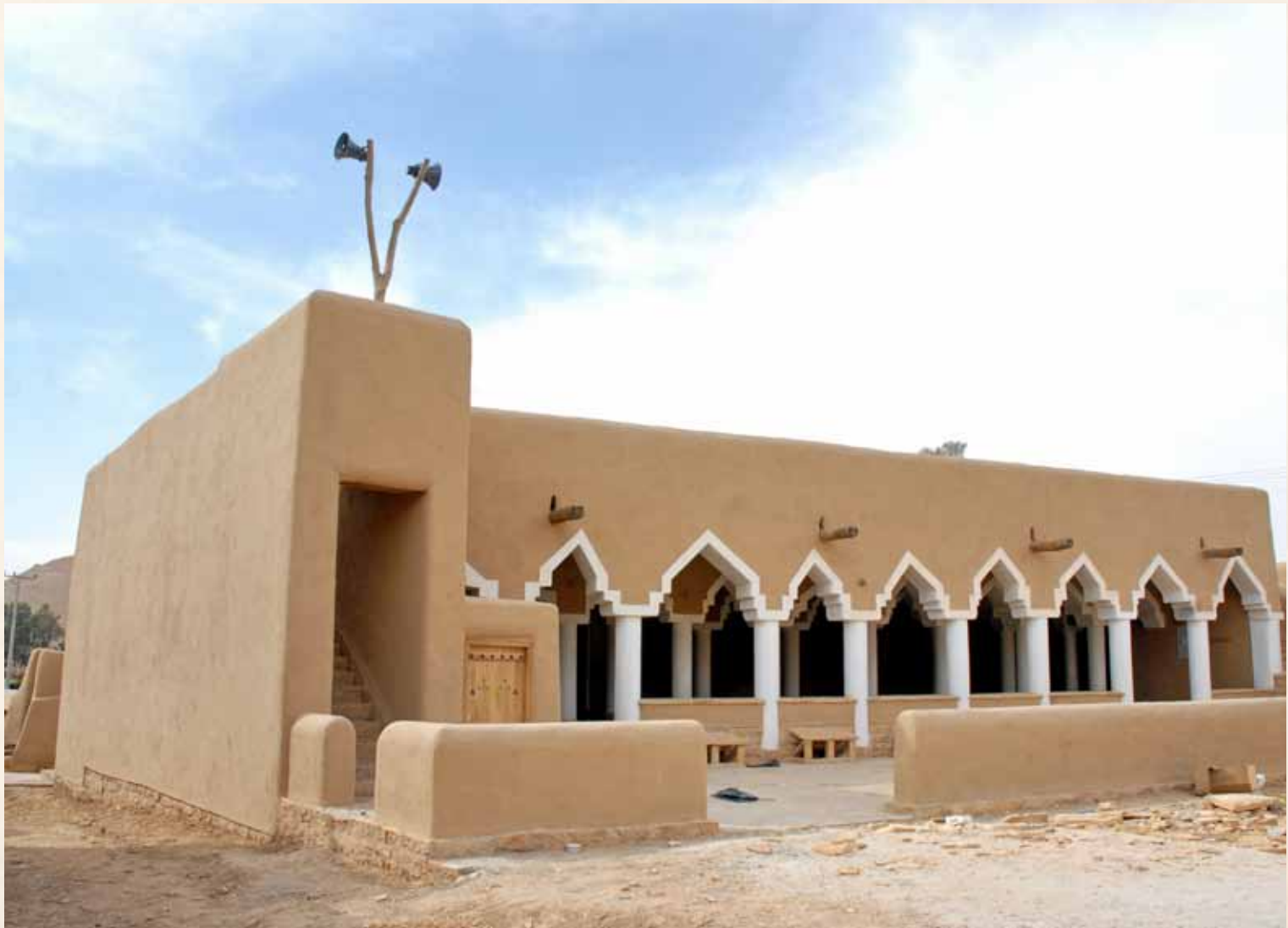
Al-Awshazah Mosque after restoration- Al-Ghat
