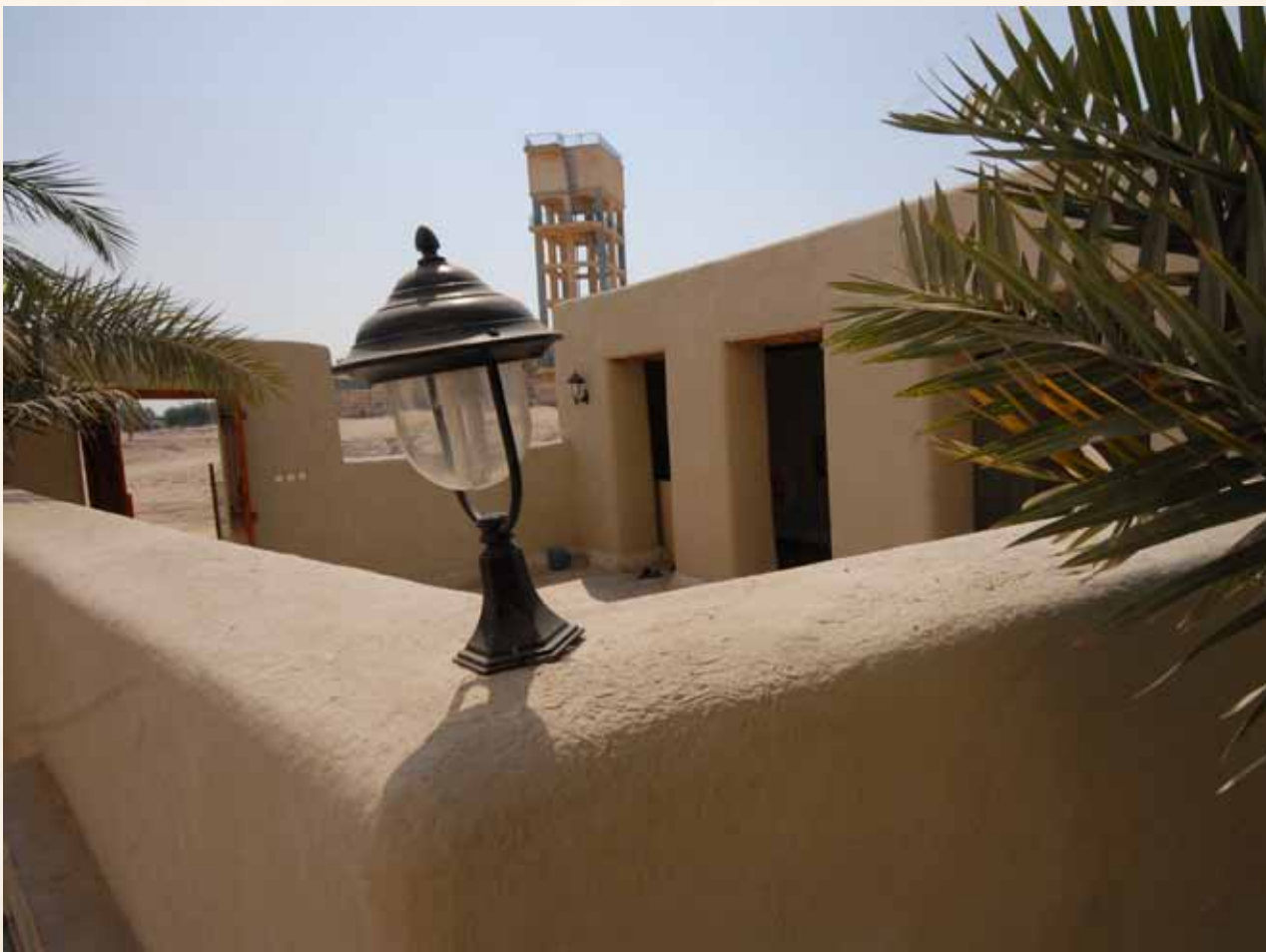
Al-Tahimiyah Mosque (2) after restoration- Tahimiyah
