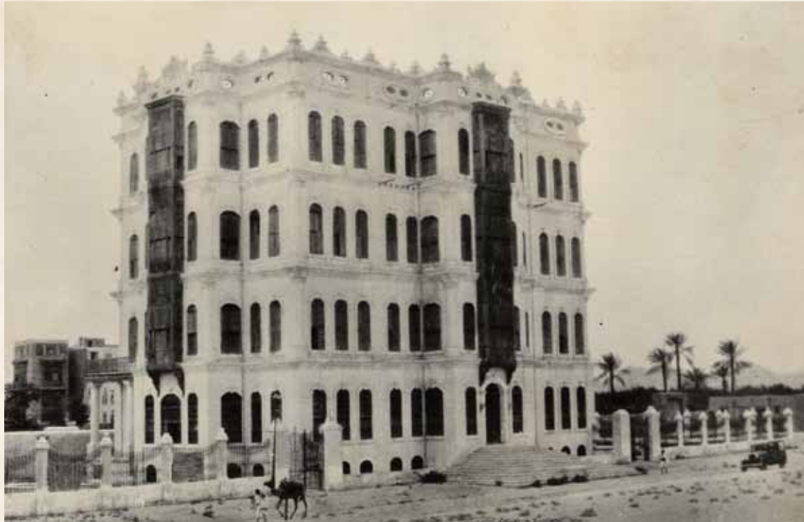
Shubra Historic Palace in Taif before restoration - Taif
