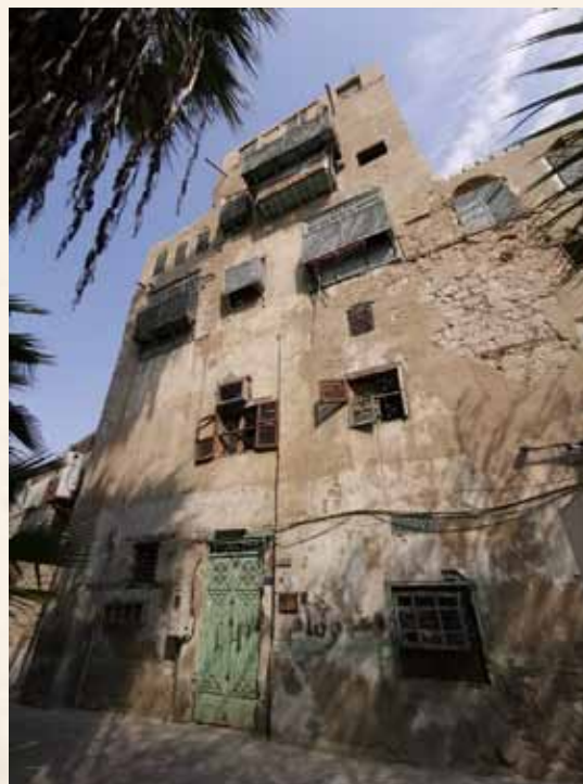
A Project to Prepare a Building Information Modeling System for Historic Buildings (HBIM) in the Historic Jeddah District (For 100 Buildings) Bayt Al Khudari
