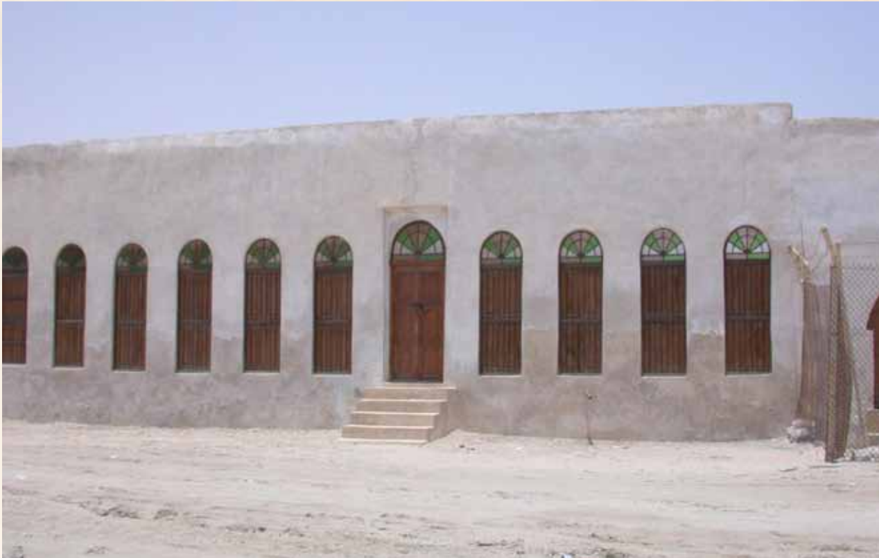
Al Uqair Mosque before restoration - Al Uqair Port, Al-Ahsa
