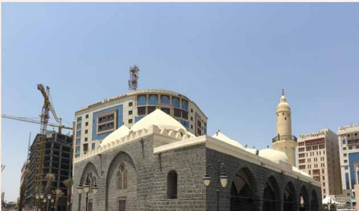
Al-Ghamama Mosque after restoration Al-Madina Al-Munawara, 1431 H (2010 AD)
