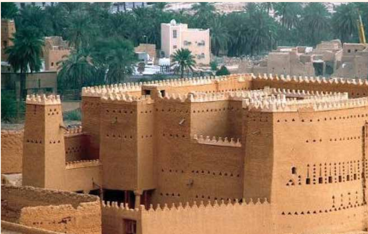
Salwa Palace Compound at Al-Taref District after restoration - Historic Ad Diriyah
