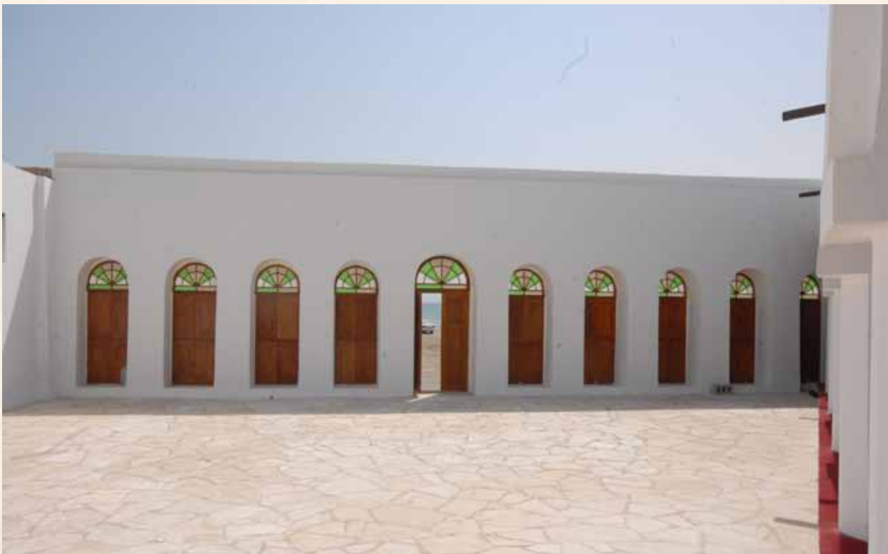
Al Uqair Mosque after restoration - Al Uqair Port, Al-Ahsa
