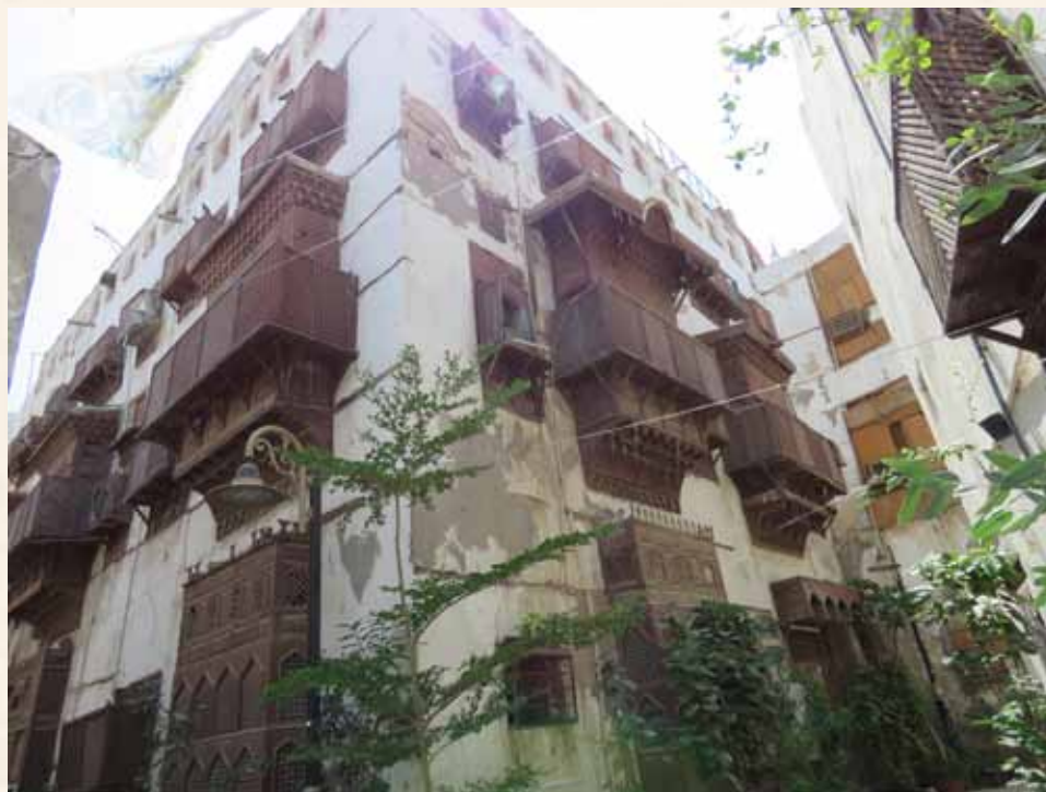
Crown Prince Project to Save and Consolidate the Historic, Archaeologic and National Listed Buildings in Historic Jeddah (56 historic buildings) Abudawood
