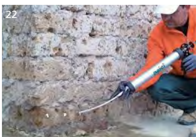
21_ Examples of injections to gravity:
