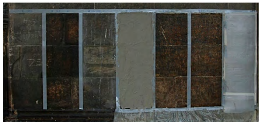
21_ Example of wrappings to clean stone surfaces.
