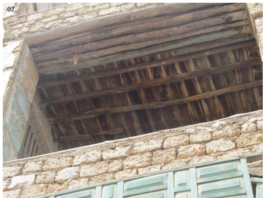
02 Architettura traditional Jeddah: masonry building with wooden floors.
