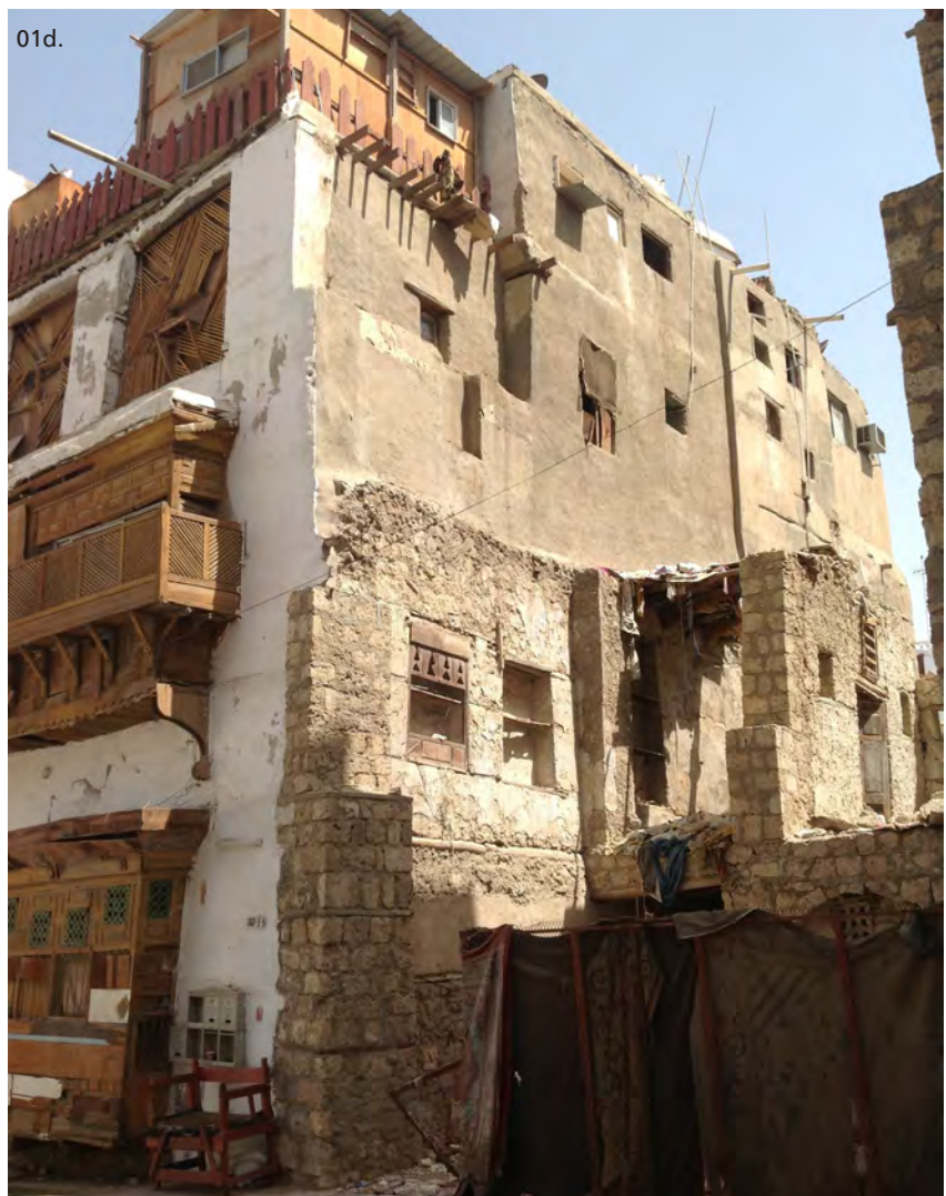
01a_01b_01c_01d_ Buildings in the historic center of Jeddah with the masonry pattern visible for the plaster detachment.
