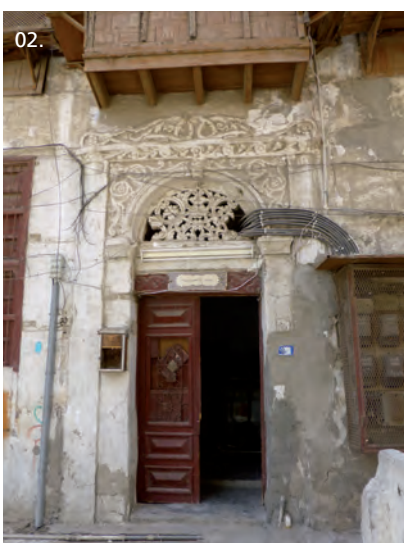
01_02 Adopted solutions for systems modernization disfigures the city, in such cases the installation has consequentially meant the demolition of the decorations.
