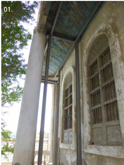
01_ Bayt Sharbatli: detail of shoring steel.
