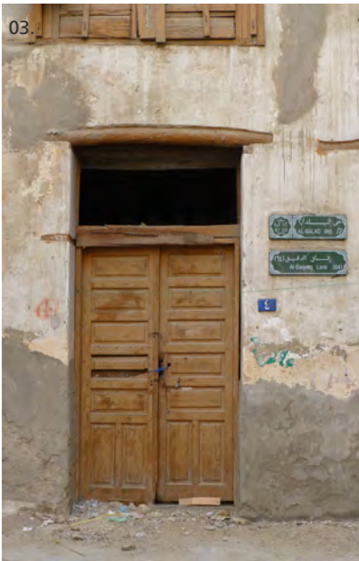
03_04_ Cement plaster applied to buildings in the center of Jeddah.
