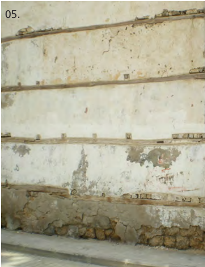
04_05_06 Deterioration caused by the rise of humidity damages the lower course of the facade affecting the plaster coating as the masonry itself.
