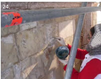
22_23_24_ Grouting operation between the stone elements.
