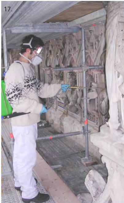
16_17_ Herbicide operation on the masonry.
